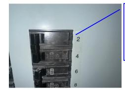
Main Panel (MPD): 40 amp breaker with #10 wires connected.
