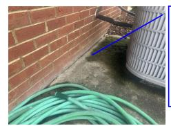
Exterior: Concrete slab for HVAC units is settled and pitched towards exterior wall.
