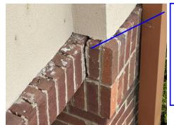
Exterior: Evidence of previous movement in brick at top side of front porch columns.
